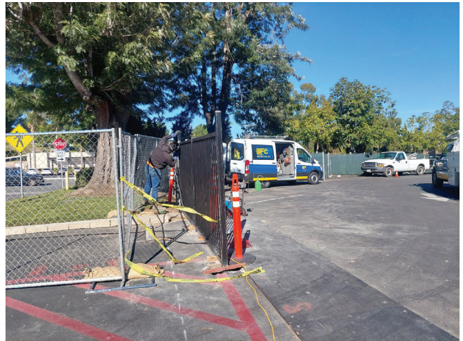
Wrought Iron Fence Installation
