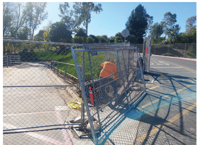
New Chain-Link Fence and Gate Installation
