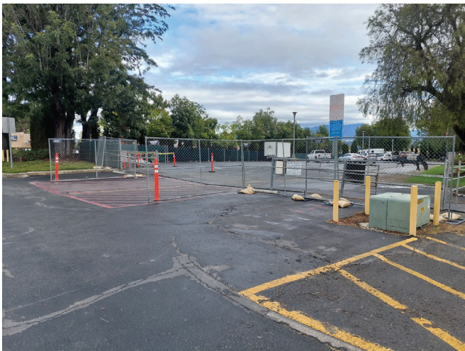
Temporary Fence and Gate
