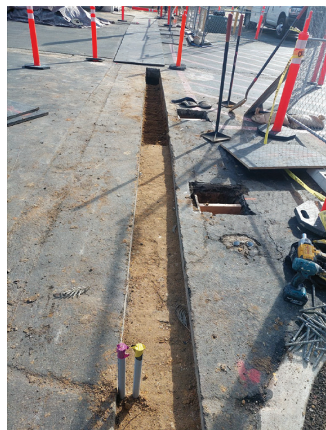
Sawcut, Excavating
